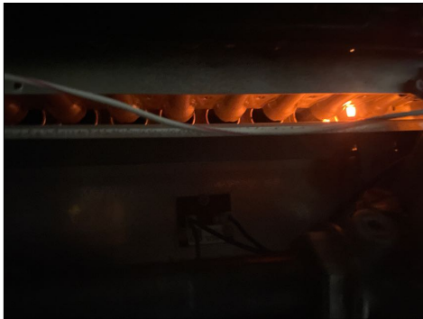
Glow plug properly activated from the thermostat at time of inspection
