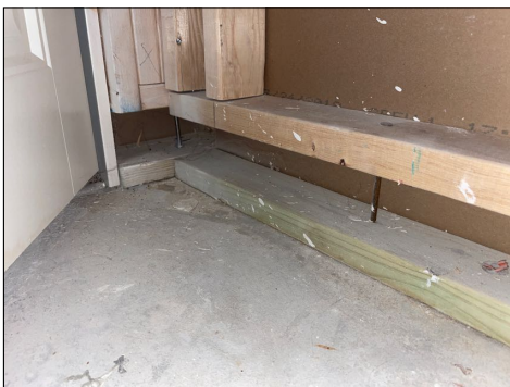
Walls are noted as properly floated
